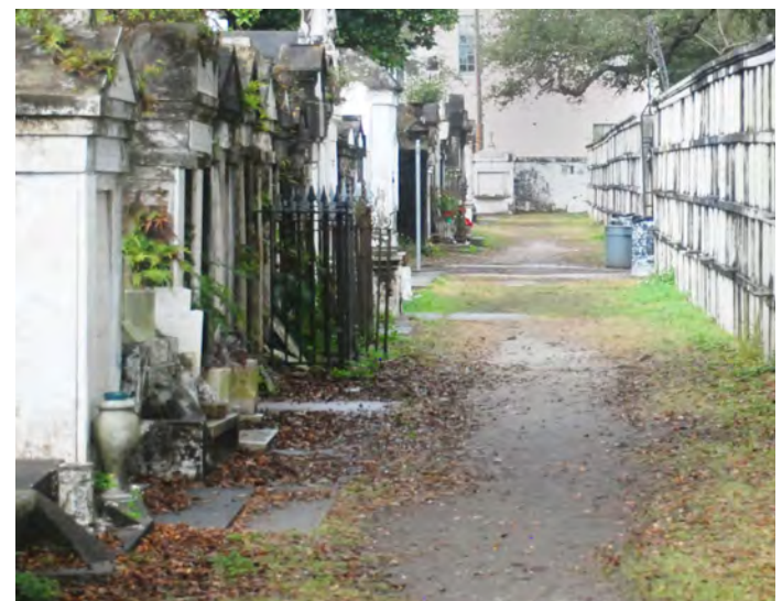
Fig. 37: Perimeter aisle parallel to Washington Avenue. Note the wall vaults on the right side.
