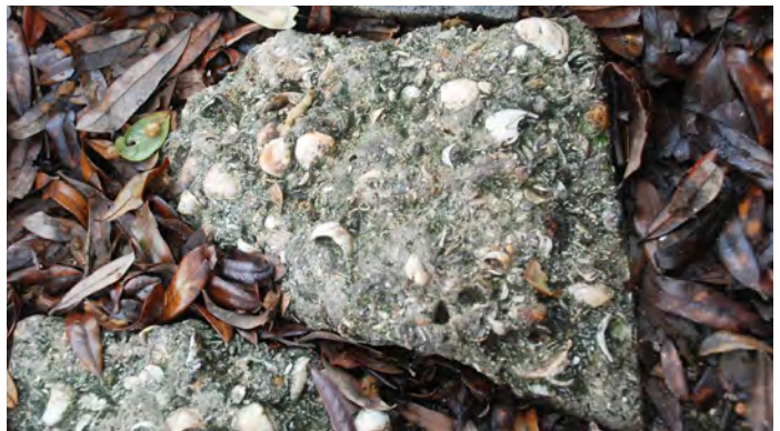
Fig. 53: Clam shells are visible in the concrete used for the Coliseum Street sidewalk. The shells, employed as aggregate, can be seen in the loose fragments of concrete that have been overturned (where the oak tree roots have cracked the sidewalk).
