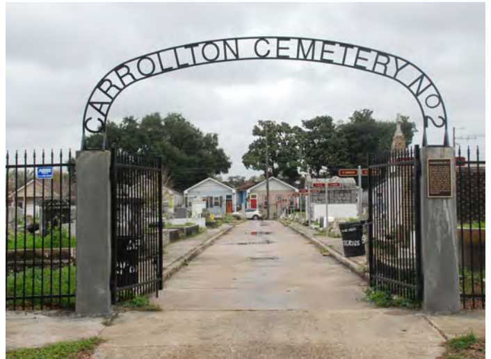
Main entrance gate
