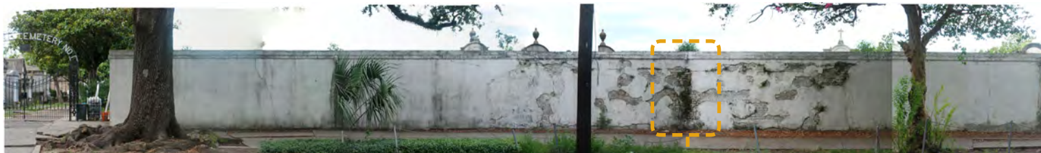
Lakeside Portion (from the main entrance gate to Prytania Street)
