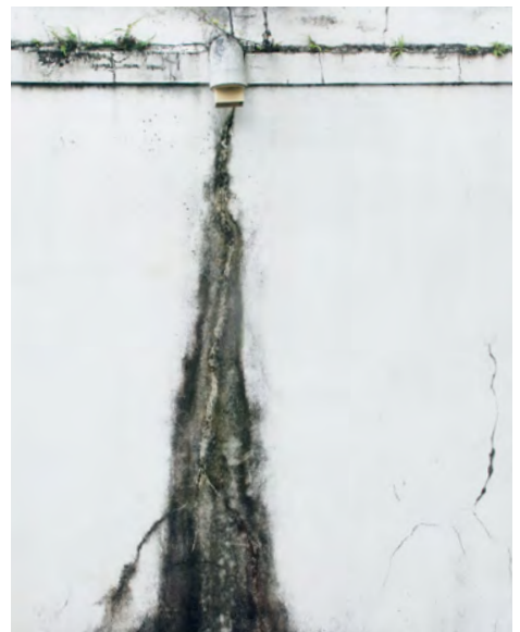
A3: The existing stucco is stained beneath one of the wall vault roof drains. Note also the cracks in the stucco surface allowing a place for moisture to enter the wall and biological growth (e.g. algae, fungi, moss, mold, lichen, plants) to form.
