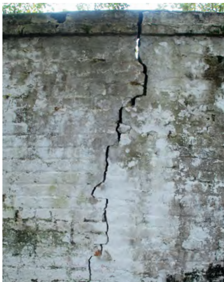
D2: A large crack has formed in this section of the wall.
