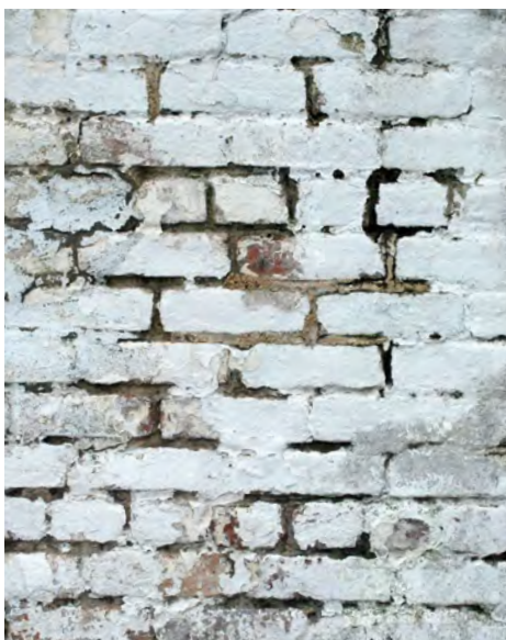
A1: Section of brick in need of repointing. The mortar is disintegrating, providing opportunities for water to infiltrate the wall.
