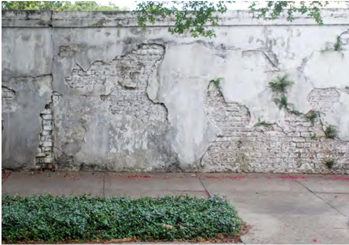
Fig. 20: Detail of the Washington Avenue wall where the cement stucco is gradually being removed
