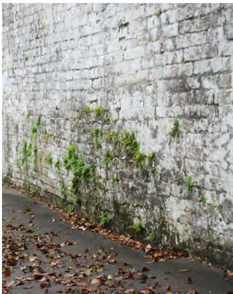
B4: The bricks in the lower portion of the wall are bulging outward. The presence of vegetation and biological growth in this area also suggests that moisture entrapment is a problem.
