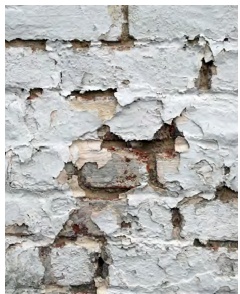
C3: Multiple coatings of paint in various shades of white are visible. The paint is flaking off, exposing weak mortar joints in need of repointing. This condition is prevalent along much of the Sixth Street wall.
