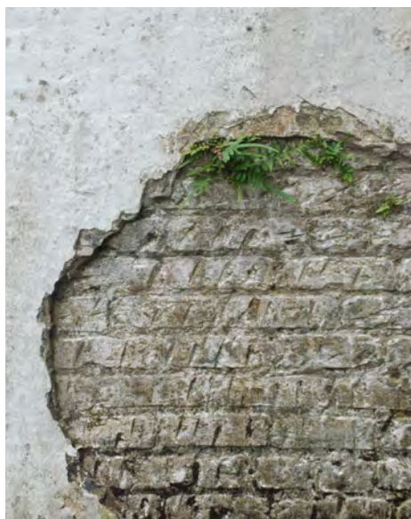
A2: The surface of the brick wall was hatched for better adhesion of the cement-based stucco (which is in now being removed in phases).
