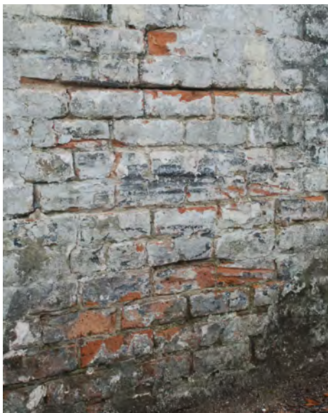
B1: Area where a car appears to have impacted the brick wall.
